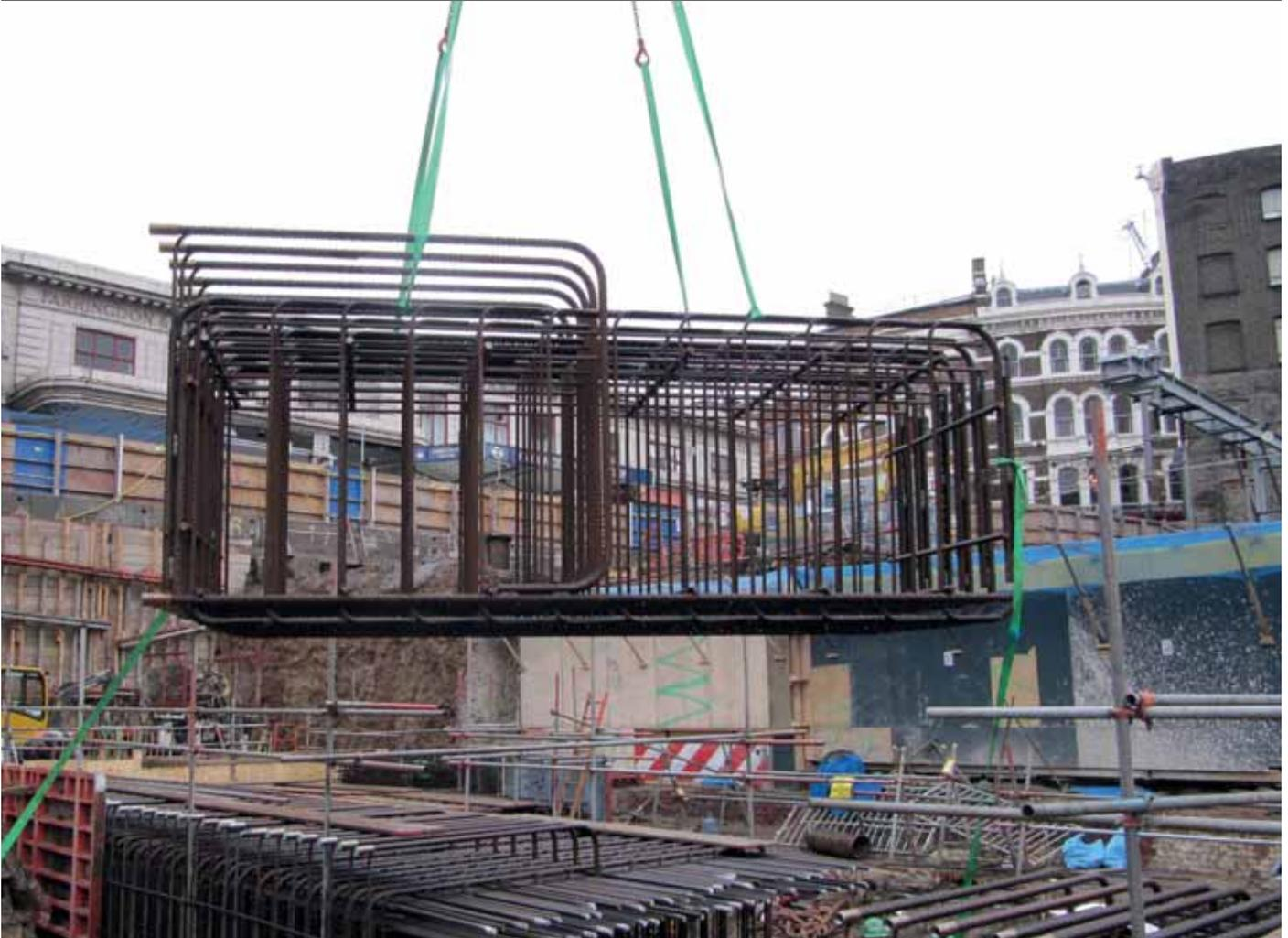
ERL Technical focuses on reducing waste and process on site by using value added products like carpet reinforcement, prefabrication and utilisation of stock lengths. Waste can be defined as anything from time to a commodity.
