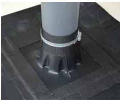
It is crucial that when gas protection is required, the site conditions, design and application are all taken into consideration to provide an impermeable membrane capable of surviving installation and subsequent traffic to protect against harmful gases. It is advisable to consider the use of pre-formed corner and cavity tray units when designing and installing gas protection membranes, especially where barriers of greater thickness are required.
